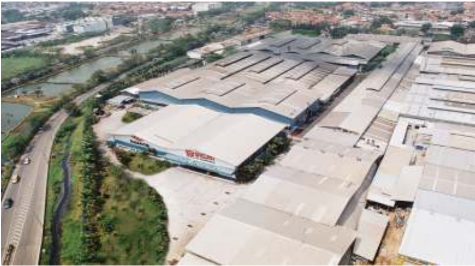
Kapuk Plant (Radiator Facilities)
